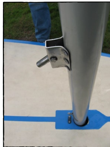
Photo 11, Insert the mast
